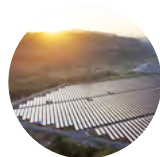
Pililla Wind Farm, Kirahon Solar Farm
